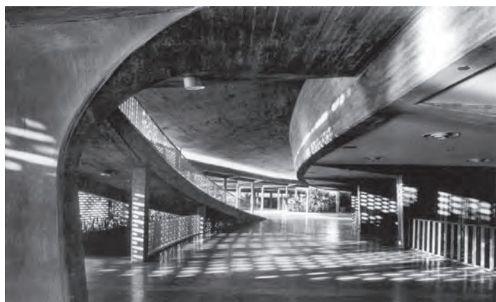
UCV, view of the Covered Plaza which the access ramp of the Aula Magna.
