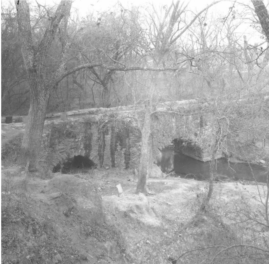
Fig. 7 – San Antonio (Texas), Mission Espada Aqueduct at the end of 19th century, photograph of Ernst Wilhelm Raba (SACS Library, San Antonio, TX). The aqueduct was described in 1772 as a conduit of lime and stone of thirty-eight varas in length, six in height with a «punta de diamante» (indicating the buttress to divert water), and «dos ojos» (or arches), which allowed the creek's currents to pass.
