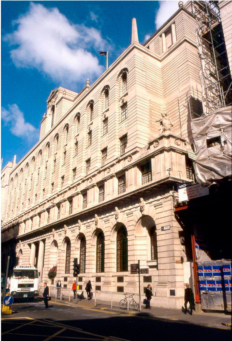
Fig.8. Midland Bank, Poultry, City of London. Headquarters Building (1924-39) by Sir Edwin Lutyens. Author's photograph.
