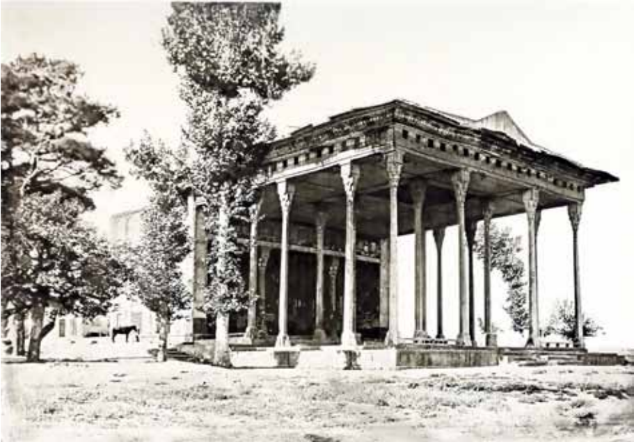
Fig. 9. Isfahan, Talar Ayene Khaneh. 9. 3. Inside view of Talar Ayene Khaneh. (P. Coste, Bibliothèque Municipale de Marseille, Ms. 1132, f. 46). 9. 4. View of Talar Ayene Khaneh. (DIEULAFOY 1884, III, pl. 6).
